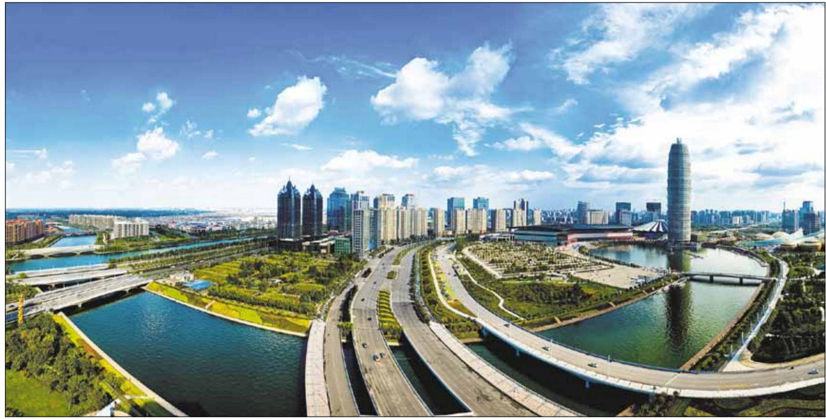
The modern development of the host city of Zhengzhou will be on display during the upcoming Expo Central China.
